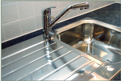
With softened water there is no hardness, no spotting and no constant cleaning!
