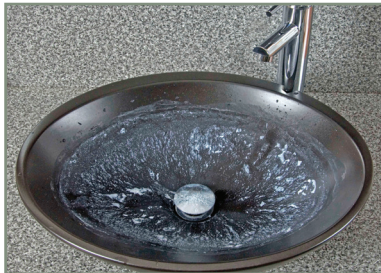
Scum is left on the surface after the water has drained away
